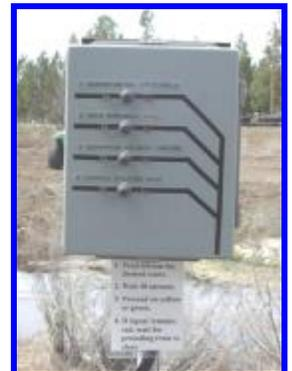
Stop by the stand and press the button for your desired route. Observe the overhead light like the one shown in the next photo and proceed when you get the required yellow or green light. When you make your selection, you do not have to worry about changing the switches under the train in front of you. The electronic switch
