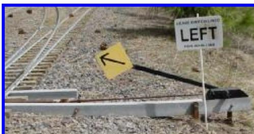
placed by the remote manual switches, but you will still find a few on the main line. To operate these switches, you simply move the arm to point in the direction you want to go. After you have moved your train through this type of switch you must realign the switch for the mainline.
