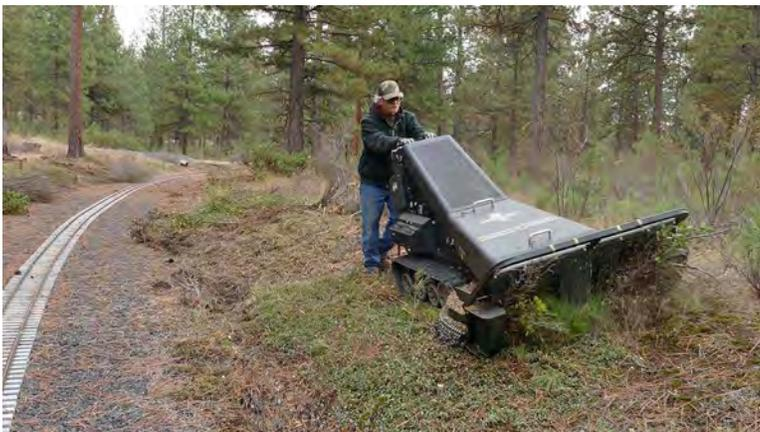
For this demonstration with the Brush Blazer, we are concentrating on increasing the visibility around corners. The further the engineer can see, the sooner the engineer can react. With all other factors being equal, the sooner the engineer can react - the sooner the train can be stopped.
