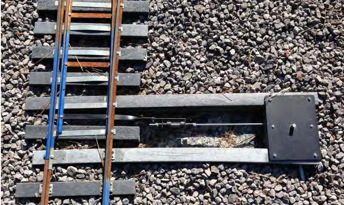
The tie without a notch located farthest from the switch stand. One with a notch located on the Switch Stand side..... so the control tube can run toward the Switch Stand. The 42" ties are positioned so the Grey Metal Box just fits between the 42" ties. Cut a hole in the plastic and dig a hole so the Grey Box will sit with its top at the level of the top of the tie.
